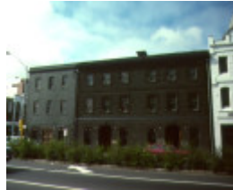
1 h66 former f blight king street
