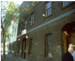
former f blight h66 exterior king street june 2001
