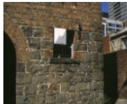
former phoenix clothing company king street melbourne detail of bluestone
