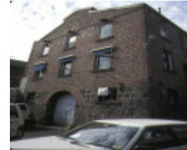
former phoenix clothing company king street melbourne rear view
