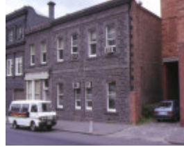
1 langdon building king street melbourne front view
