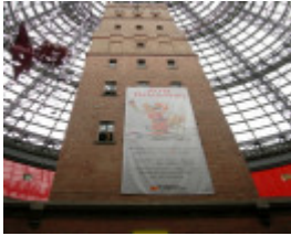
COOPS SHOT TOWER AND FLANKING BUILDING SOHE 2008
