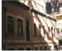
coops shot tower & flanking building knox place melb front view
