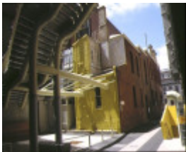
former foresters hall la trobe street melbourne rear view dec1997
