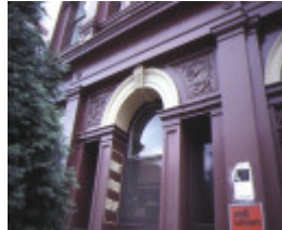
former foresters hall la trobe street melbourne entrance detail sep1980
