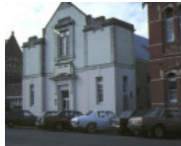
school of mines ballarat former church
