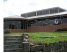
Building G, E J T Tippett Building.jpg
