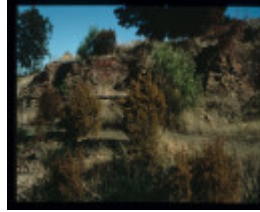
CALEDONIAN CRUSHING MILL
