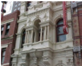
sum kum lee little bourke street melbourne balcony detail jul1999
