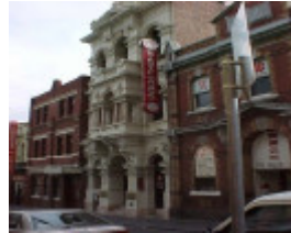
sum kum lee little bourke street melbourne front view jul1999
