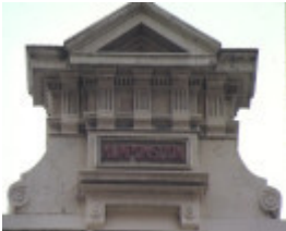
num pon soon little bourke street melbourne detail parapet
