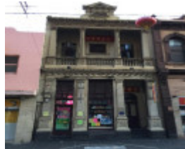
NUM PON SOON SOCIETY BUILDING July 2016
