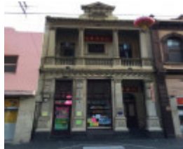
NUM PON SOON SOCIETY BUILDING July 2016
