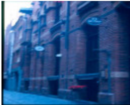
h00473 warehouses niagara lane3
