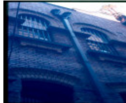
h00473 warehouses niagara lane2
