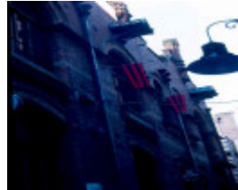
h00473 warehouse niagara lane
