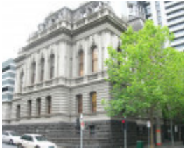
FORMER RECORDS OFFICE SOHE 2008
