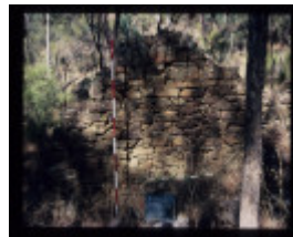
BATTERY SITES: EUREKA CO & PHOENIX CO FEATURE
