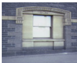
bank of nsw queen street melb exterior window detail
