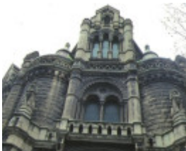
magistrates court russell street melbourne entrance elevation
