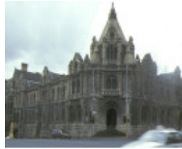
magistrates court russell street melbourne front view
