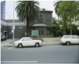
police garage russell street melbourne view of side of building
