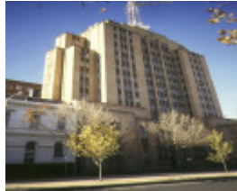
1 police headquarter's complex russell street melbourne front elevation jun1997
