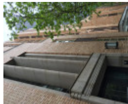
POLICE HEADQUARTERS COMPLEX Nov 2016
