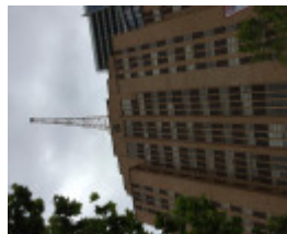
POLICE HEADQUARTERS COMPLEX Nov 2016
