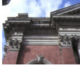
former church of christ stanton street abbotsford pediment detail sep1985
