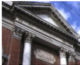
former church of christ stanton street abbotsford pediment sep1985
