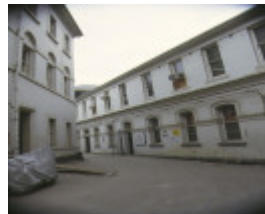
treasury reserve precinct spring street st andrews place & treasury place side elevation paper store 1997
