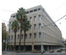
Former State Chemical Laboratoires Treasury Precinct, April 2012.JPG
