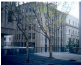
Treasury Reserve Precinct Western Annex Demolished
