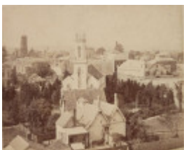
Bowling Green site: St Peter's and manse
