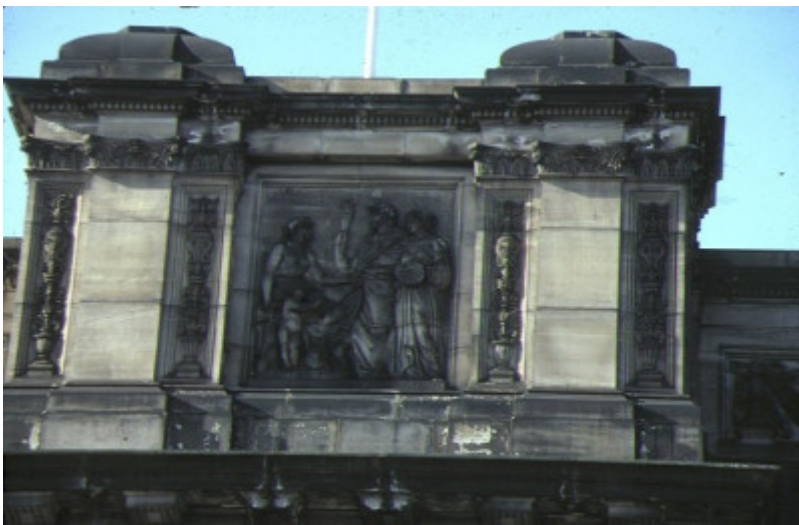
parliament house grounds works & fences spring street melbourne relief detail
