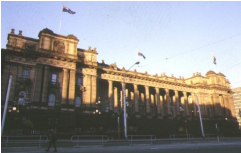
1 parliament house grounds works & fences spring street melbourne front view
