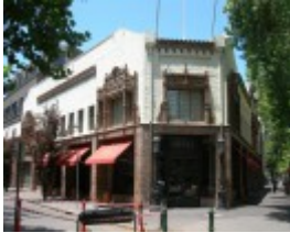
FORMER KELLOW FALKINER SHOWROOMS SOHE 2008
