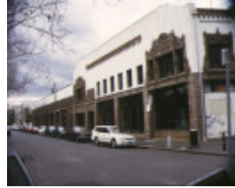
1 former kellow falkiner showrooms st kilda road melbourne front view
