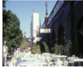
1 princes walk vaults batman avenue melbourne cafes on walk feb1985
