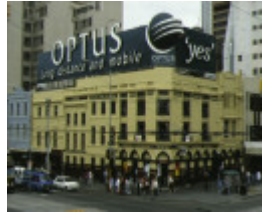
1 young & jackson's princes bridge hotel swanston street melbourne corner view
