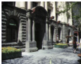
melbourne town hall swanston street melbourne ext bluestone
