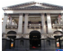
H0001 melbourne town hall and administration bldg swanston street melbourne main entrance she project 2004
