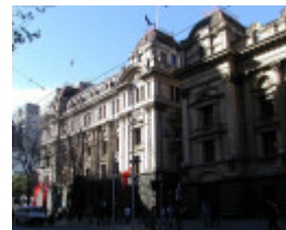
H0001 melbourne town hall and administration bldg swanston street melbourne front she project 2004
