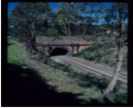
ELPHINSTONE RAILWAY TUNNEL
