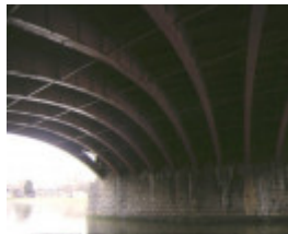
princes bridge over yarra river melbourne underside sep1998
