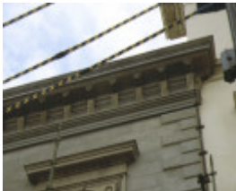
anz bank ballarat roof detail
