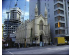
1 john knox free presbyterian church swanston street melbourne front elevation
