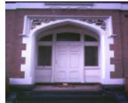
residence sturt street ballarat front entrance
