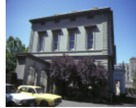
1 former royal mint williams street melbourne side view feb1985
