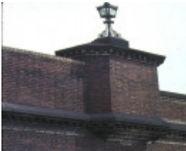
former royal mint williams street melbourne light on surrounding wall
