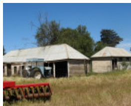
Exford stable buildings
