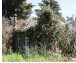
Exford west pavilion
