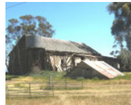
Exford barn & underground tank
