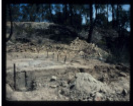
MORNING LIGHT MINE EXCAVATION
