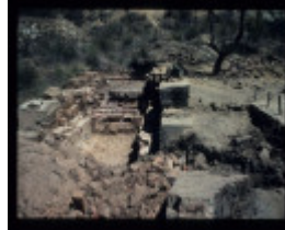
MORNING LIGHT MINE EXCAVATION
