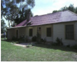
1 koonoona merricks road merricks north front view homestead
