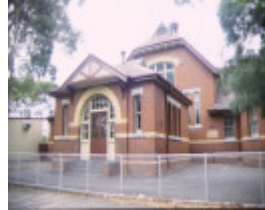
1 primary school no 2815 richardson street middle park infant school front view feb1998
