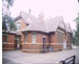
primary school no 2815 richardson street middle park infant school side view feb 1998
