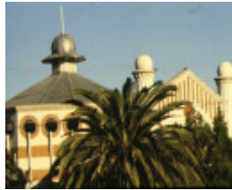
methodist church cnr deakin avenue & tenth street mildura view of roof line jun1980
