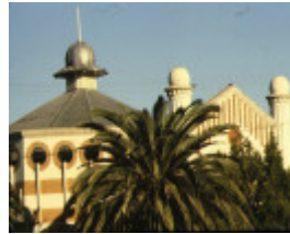
methodist church cnr deakin avenue & tenth street mildura view of roof line jun1980
