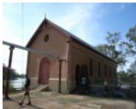
PSYCHE BEND PUMPING STATION SOHE 2008
