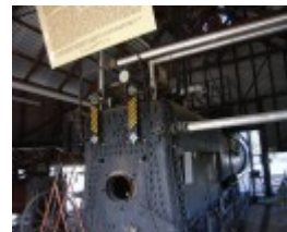
PSYCHE BEND PUMPING STATION SOHE 2008
