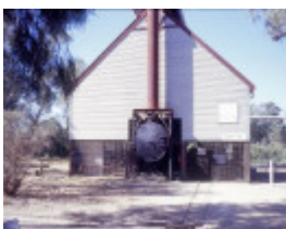
h00548 psyche bend pumping station psyche bend mildura smoke box and chimney base she project 2003
