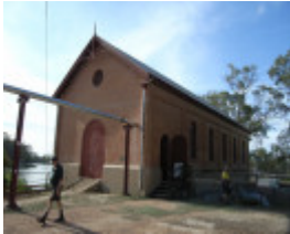
PSYCHE BEND PUMPING STATION SOHE 2008
