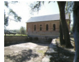
1 psyche bend pumping station psyche bend mildura rear view
