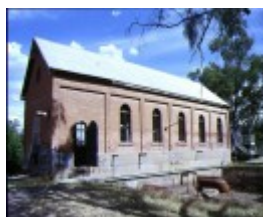
psyche bend pumping station psyche bend mildura front view dec1990
