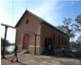
PSYCHE BEND PUMPING STATION SOHE 2008
