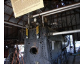
PSYCHE BEND PUMPING STATION SOHE 2008
