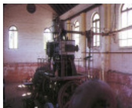
psyche bend pumping station psyche bend mildura interior with machinery
