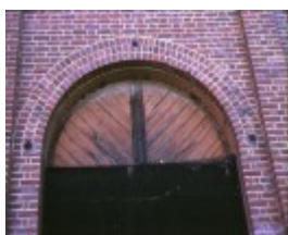
psyche bend pumping station psyche bend mildura detail entrance
