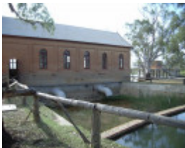
PSYCHE BEND PUMPING STATION SOHE 2008
