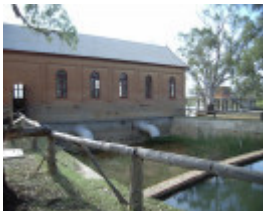
PSYCHE BEND PUMPING STATION SOHE 2008
