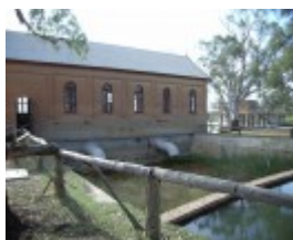
PSYCHE BEND PUMPING STATION SOHE 2008
