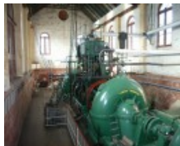
PSYCHE BEND PUMPING STATION SOHE 2008
