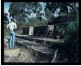
NEW NAPOLEAN MINE BATTERY
