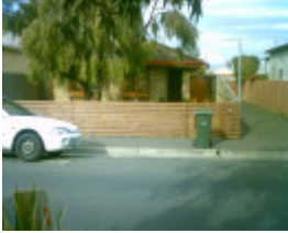
19 O'Connell Street, Geelong West
