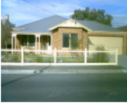
25 O'Connell Street, Geelong West
