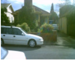
28 O'Connell Street, Geelong West
