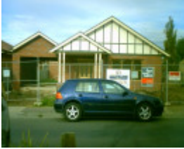
43 O'Connell Street Geelong West
