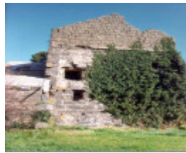
bluestone mill mill street mortlake end wall aug1993
