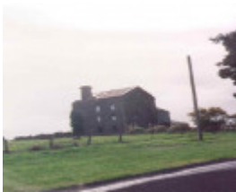
bluestone mill mill street mortlake front view aug1993
