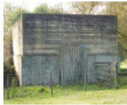
Concrete silage store from west 2017.jpg
