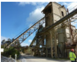
Picking station and incline hoist from grarry from east 2017.jpg
