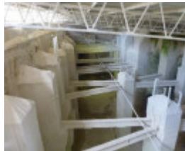
Tunnel from north 2017.jpg
