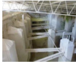
Tunnel from north 2017.jpg
