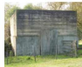
Concrete silage store from west 2017.jpg
