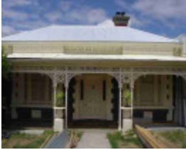
richmond waltham street richmond waltham street 29
