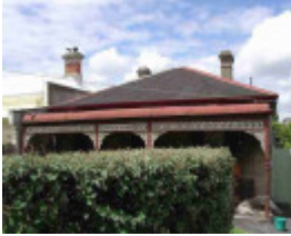
richmond waltham street richmond waltham street 31
