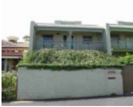
richmond richmond terrace richmond richmond terrace 85 unit 1
