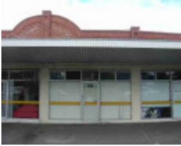
carlton north park street carlton north park street 326
