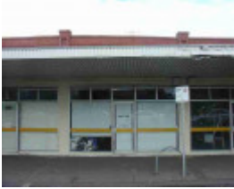
carlton north park street carlton north park street 328
