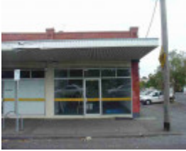
carlton north park street carlton north park street 330
