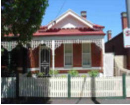
carlton north park street carlton north park street 444
