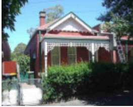
carlton north park street carlton north park street 454
